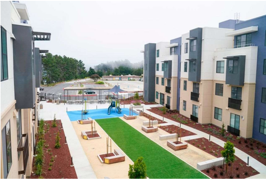
A view of a new housing complex for Jefferson Union High School District teachers and education staff in Daly City, California.
